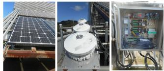
Fig. Photovoltaic modules (left), meteorological instruments (middle), and data acquisition systems (right) installed in Kagoshima Prefectural Institute of Industrial Technology.
